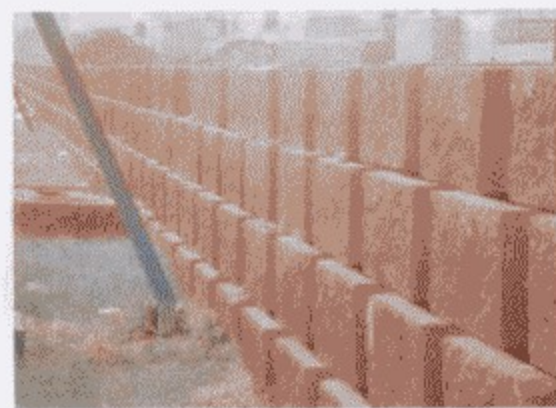
图2-51 预制混凝土砌块挡土墙
